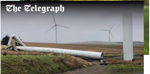
Tower-joint failure..?!!
